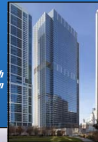
300 East Randolph Vertical Completion
